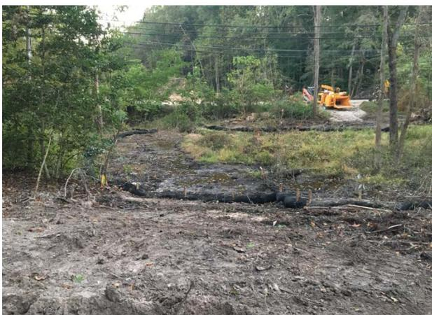
Photo 5 – Clearing and filter logs north of West Benfield Rd
