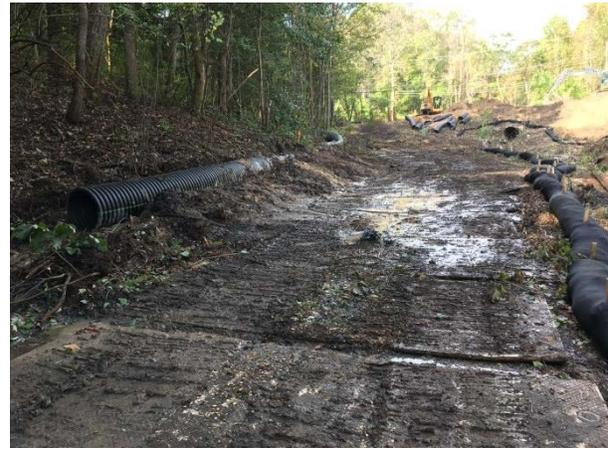
Photo 4 – Diversion pipe, mats, and filter logs south of West Benfield Rd
