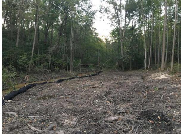
Photo 6 – Clearing and filter logs north of West Benfield Rd
