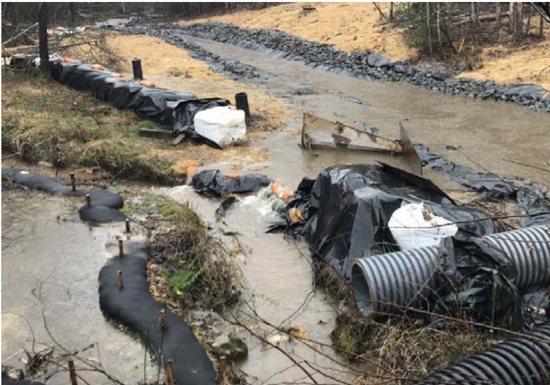
Photo 3 – Water overflowing the diversion channel & flooding the work area
