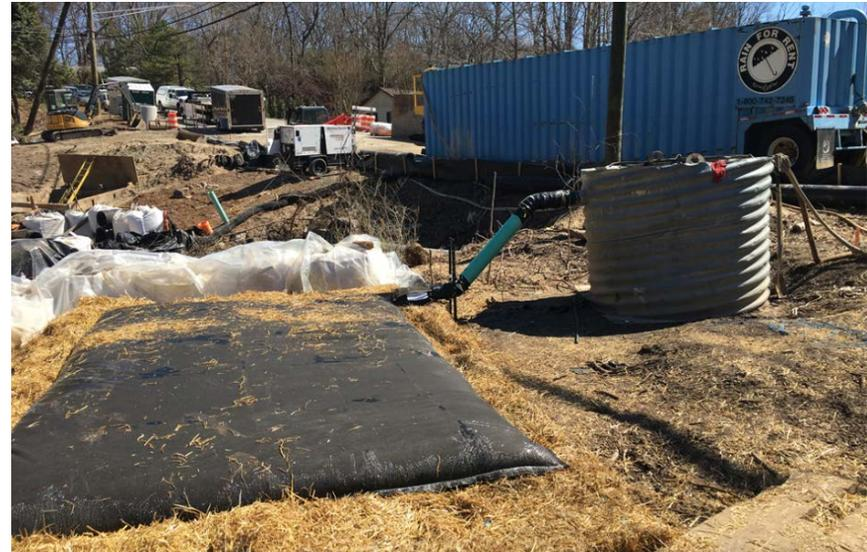
Photo 4 – Filter bag and Water Tank used to reduce turbidity
