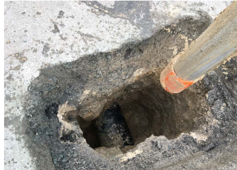
Photos 3 & 4 – A Vacuum Truck is used to remove soil and locate existing underground utility lines.
