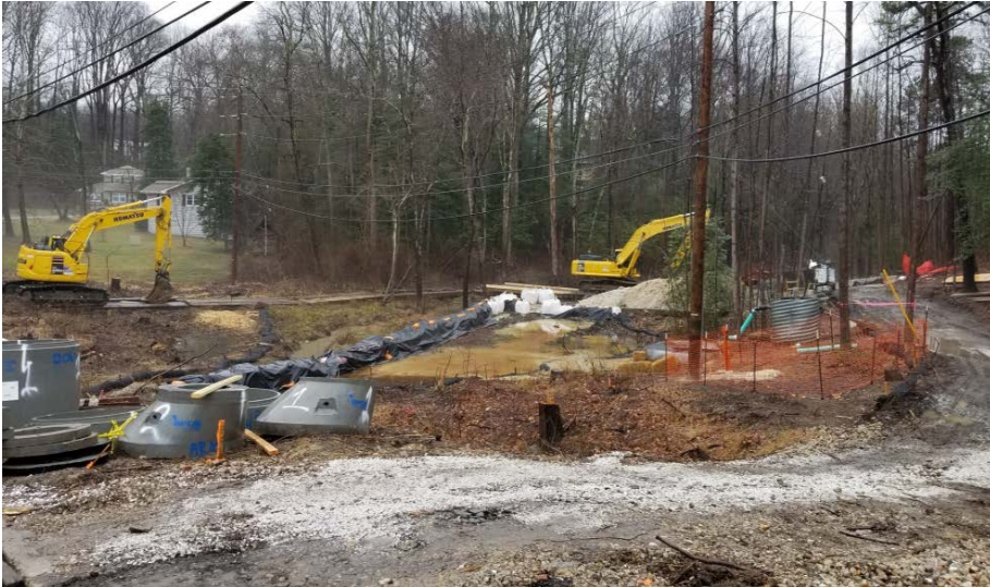
Photo 1 – Muddy conditions as sanitary sewer manholes are installed. Photo 2 – Sanitary sewer installation w/ rebar for concrete encasement
