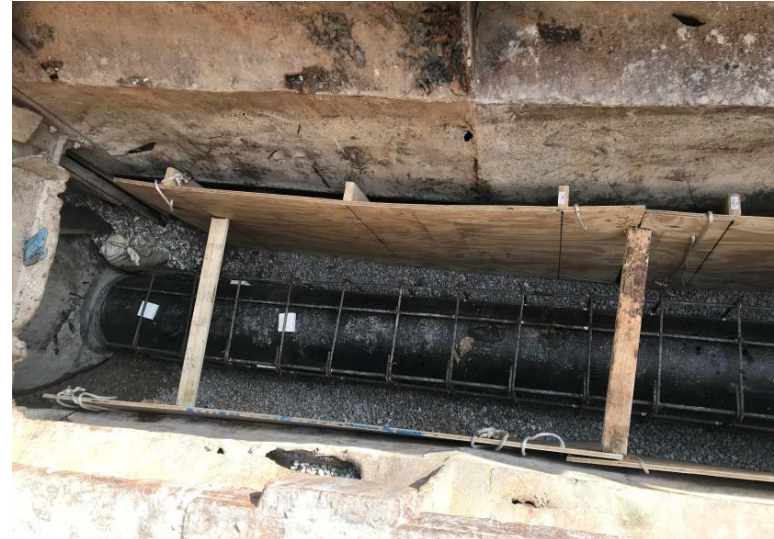
Photo 1 – Muddy conditions as sanitary sewer manholes are installed. Photo 2 – Sanitary sewer installation w/ rebar for concrete encasement
