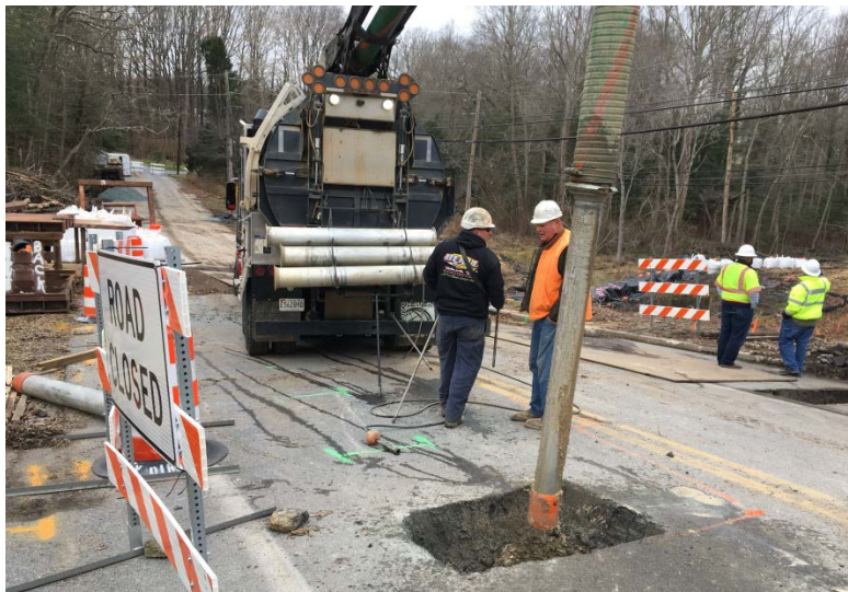
Photos 3 & 4 – A Vacuum Truck is used to remove soil and locate existing underground utility lines.
