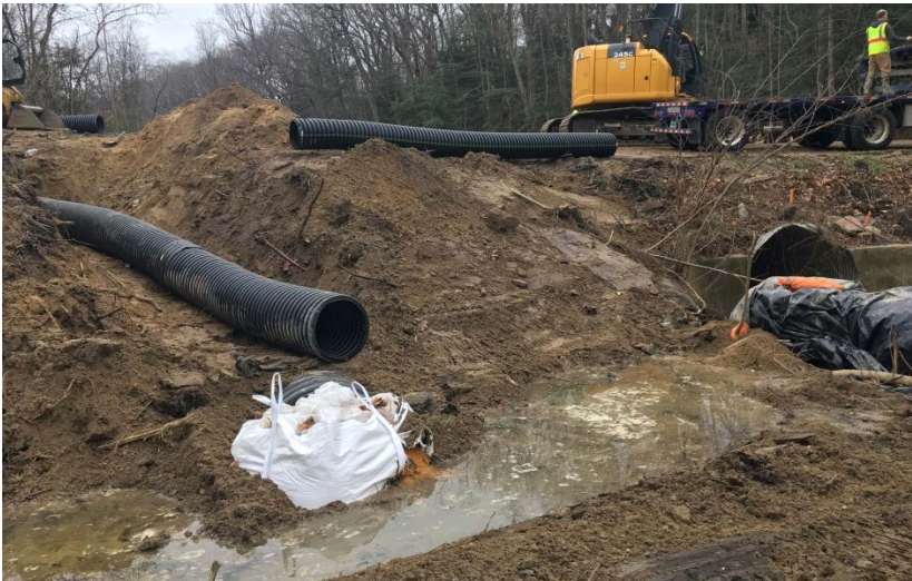
Photo 3 – Diversion pipes to left and existing culvert to right
