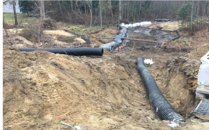
Photo 2 – Diversion pipe installation after utility pole removal
