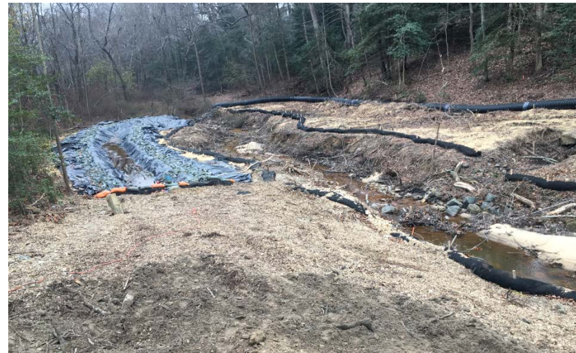
Photo 4 – View downstream of West Benfield Road: Stream diversion channel to left, existing stream to right
