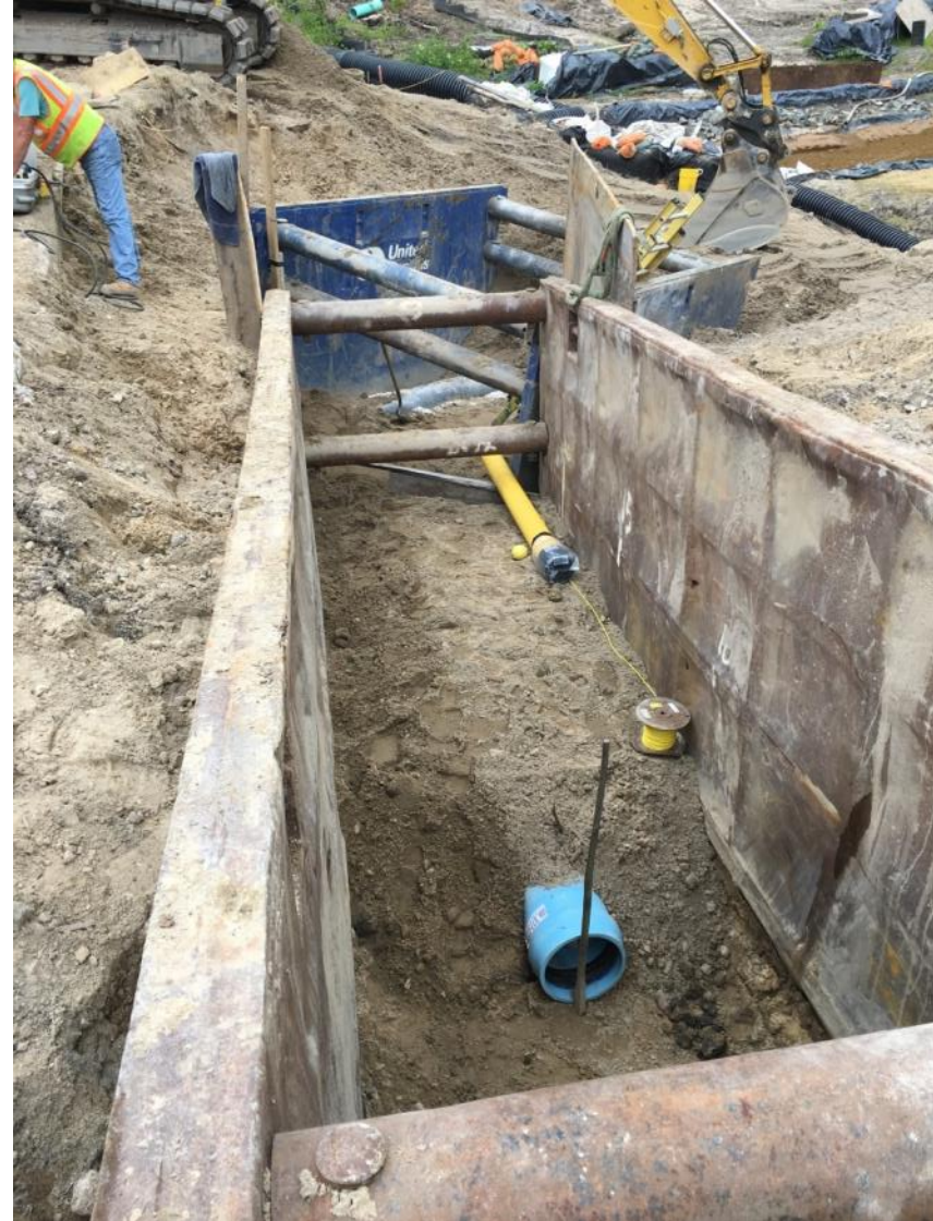
Photos 3 & 4 – Installation of the utility bypass lines
